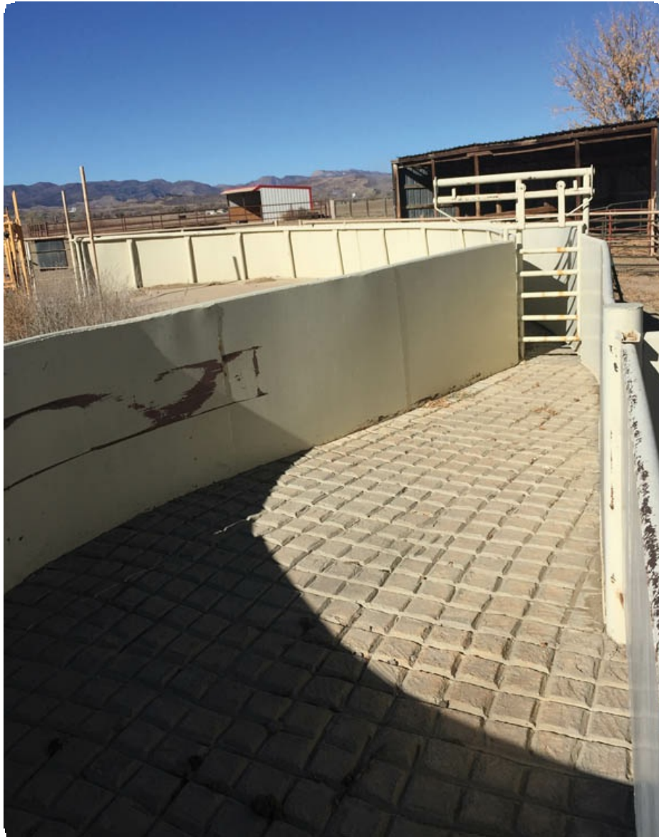
ABOVE: Deep-grooved concrete floors (from GrandinLivestockHandlingSystems.com )
